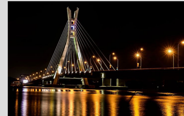
5 MINS - LEKKI-IKOYI LINK BRIDGE
